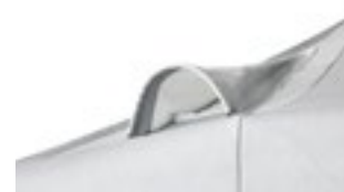
Dormers on the roof allow the smoke to escape.
